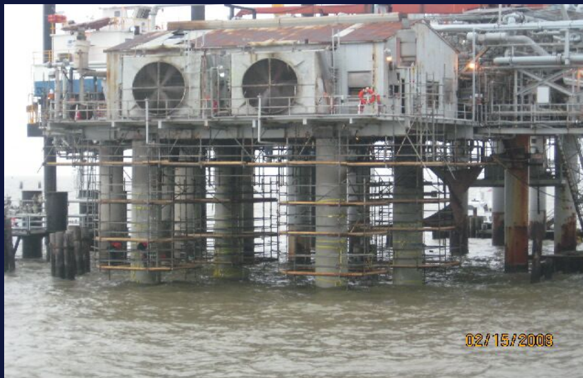
Scaffolding in place & SCR Type 1 encapsulation in progress.
