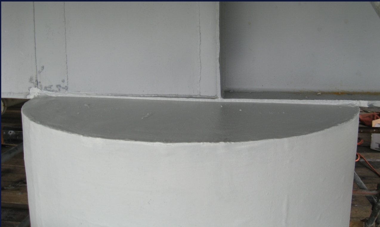
MADCON SCR Type 1 Repair (FRP with Epoxy Grout ) with Carbon Fiber & Finish Coat of Paint
