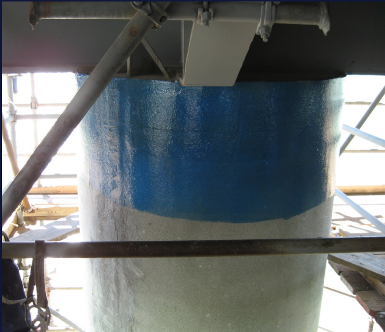
Fiberglass jacket with adhesive saturant applied prior to carbon fiber. Fiberglass jacket is filled with epoxy grout.
