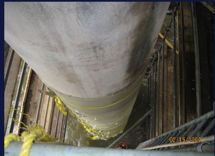
Piling with some of fiberglass in place for encapsulation.
