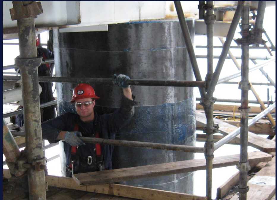
Second layer carbon fiber applied over fiberglass.
